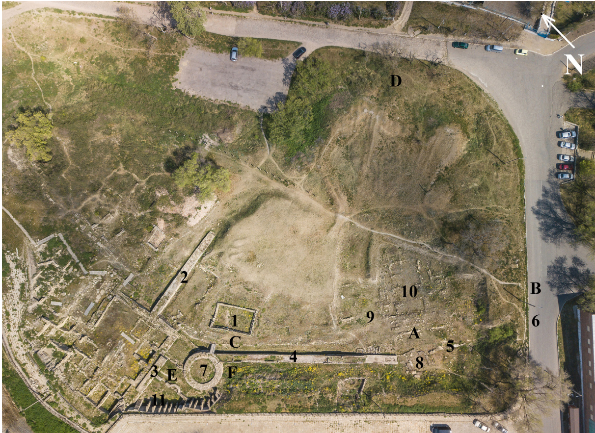
Fig. 1. Roman citadel in Tyras (drone snapshot taken by O. Hymanov 2020, modified by the author 2023). 1 – vexillation building; 2-5 – fragments of defensive walls; 6 – location of discovery of a fragment of a defensive wall; 7-8 – defensive towers; 9 – location of construction no. 497; 10 – monumental building with porticoes (structure no. 702); 11 – building with an apse (room no. 610);
