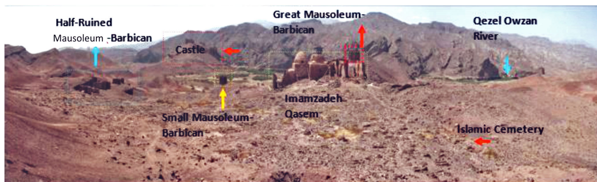
Fig. 5. Location of the Semiran site structures.
