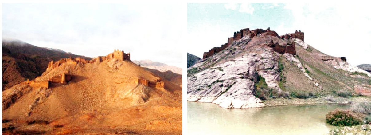
Fig. 1. Semiran Castle, view from the south and north-west.
